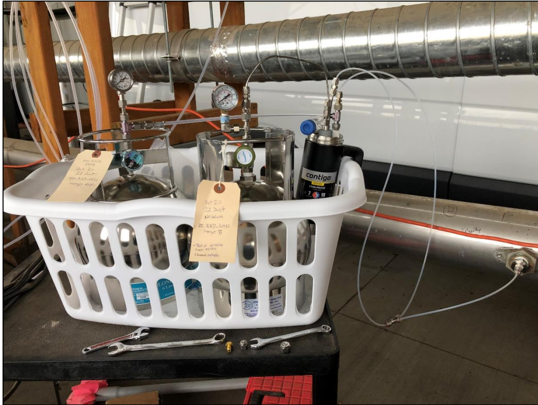
Side by side sampling from duct
